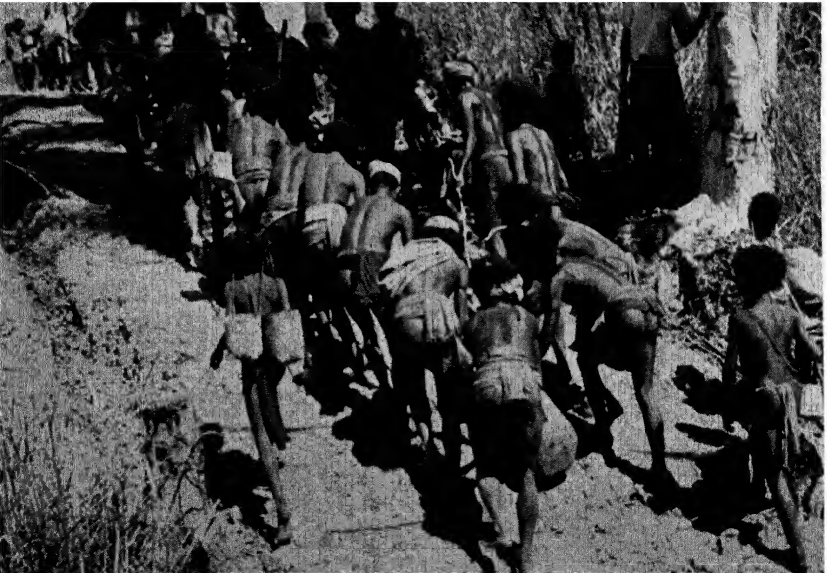
Pulling in a floor beam.
